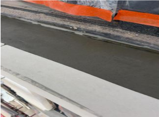
A photo Concrete repairs to stone work
