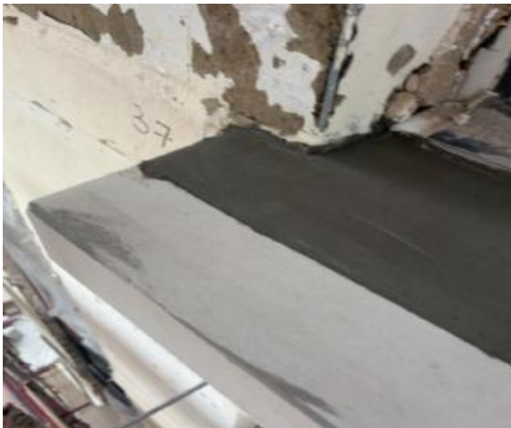
A photo Concrete repairs to stone work
