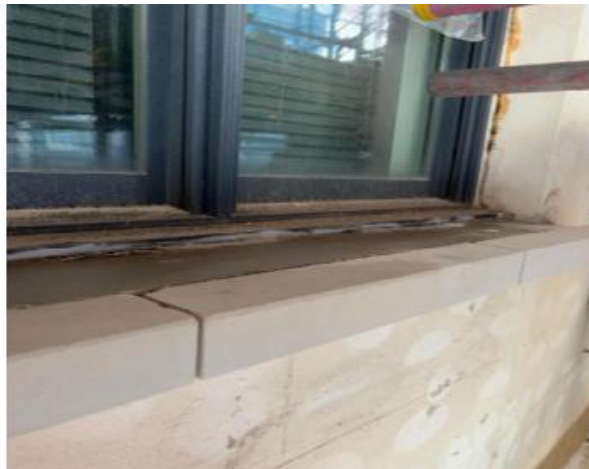
A photo Concrete repairs to stone work
