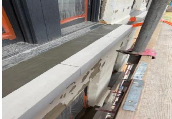
A photo Concrete repairs to stone work
